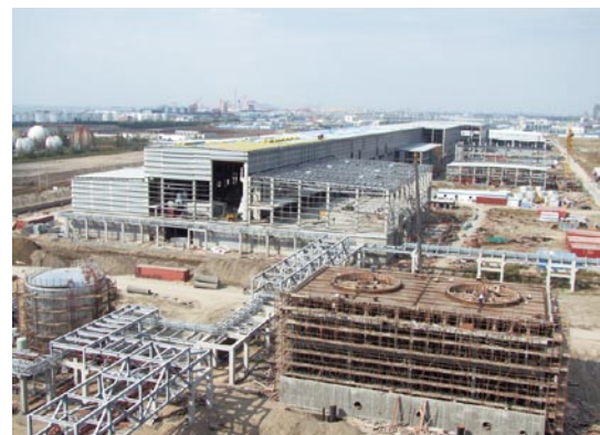
The Nantong Mill under construction
