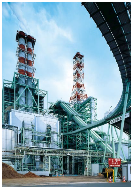
New energy boiler at Oji Paper's Yonago Mill
